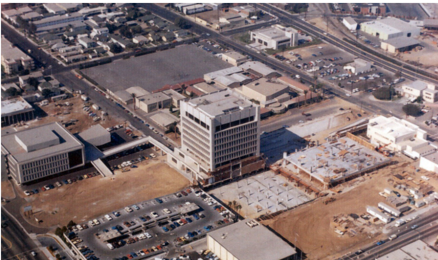
Top Photo: Construction - Inglewood Public Library Collection
